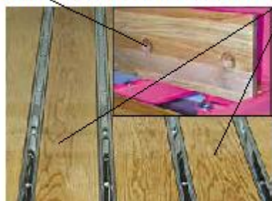
bolts through bed sills only-dome bottom of boards- for the clean floor look
